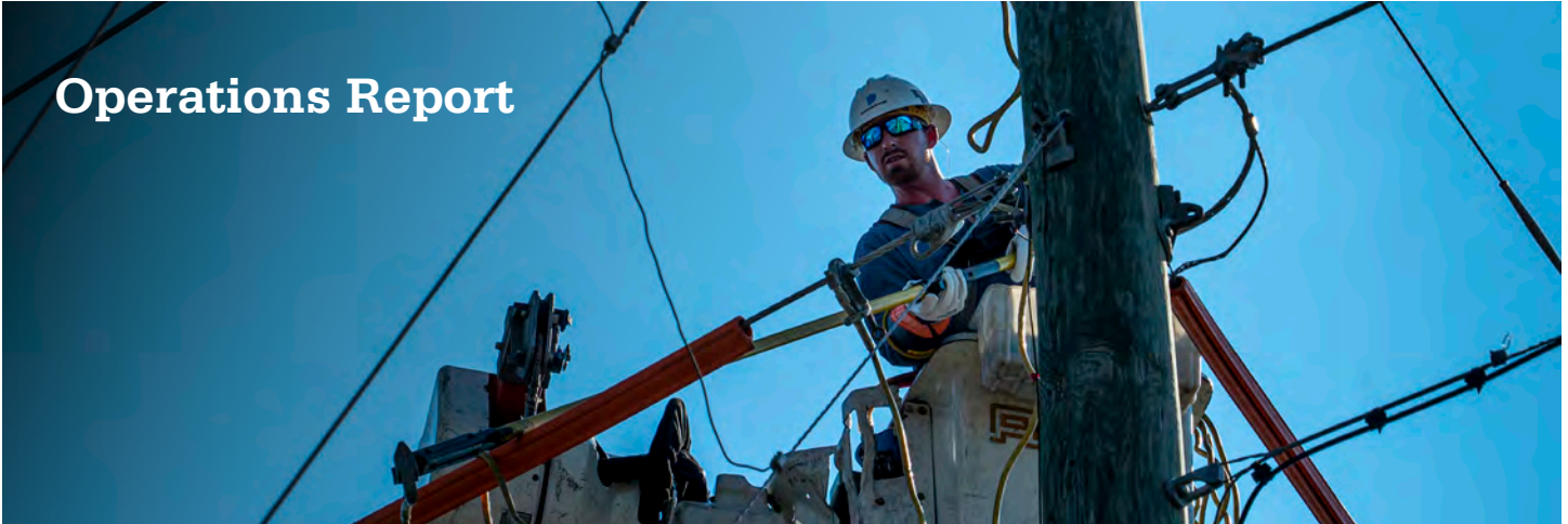
Dominion Energy Lineman; Charleston, SC
