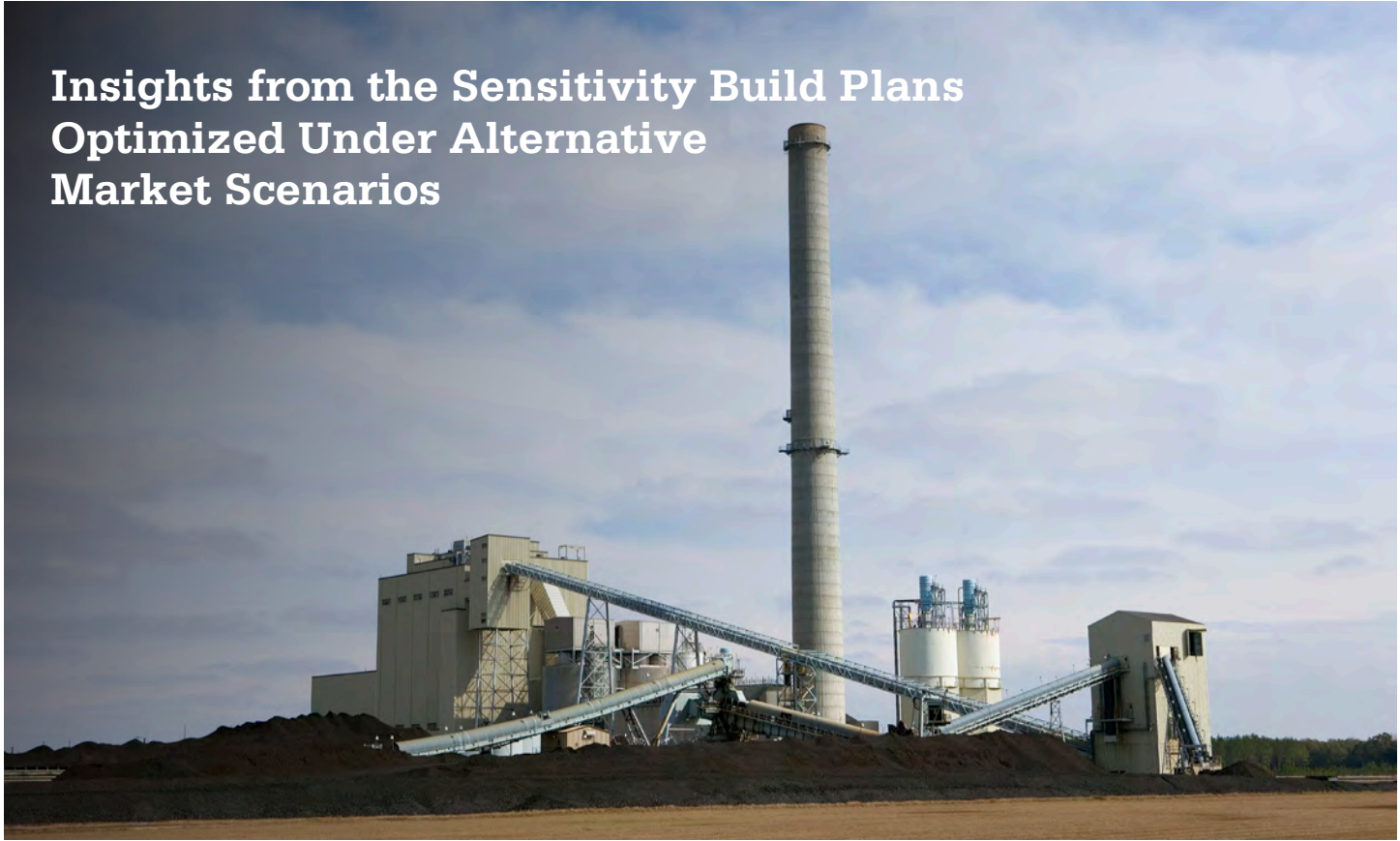
Cope Station; Cope, South Carolina
