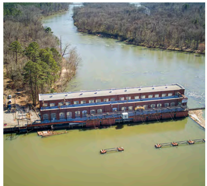
Parr Hydro Station; Farifield County, SC
